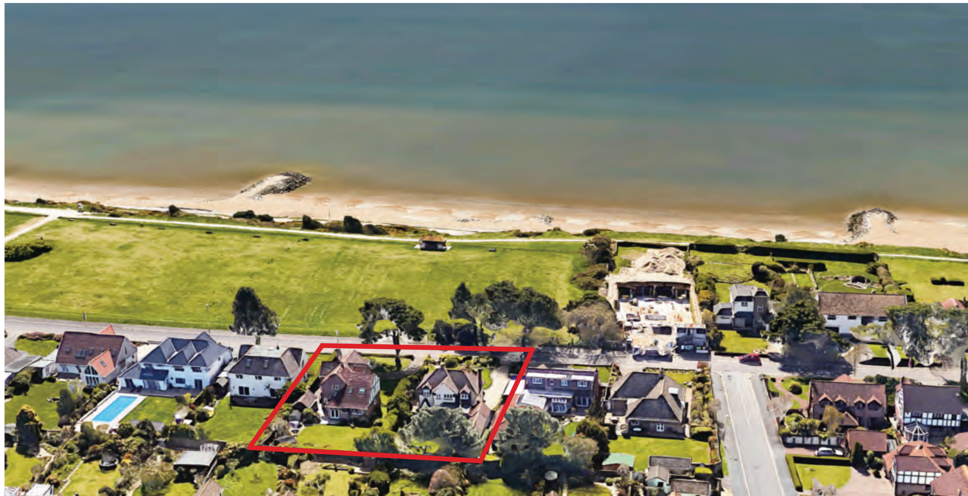
Site prior to demolition and construction of Azzurra & Luna
